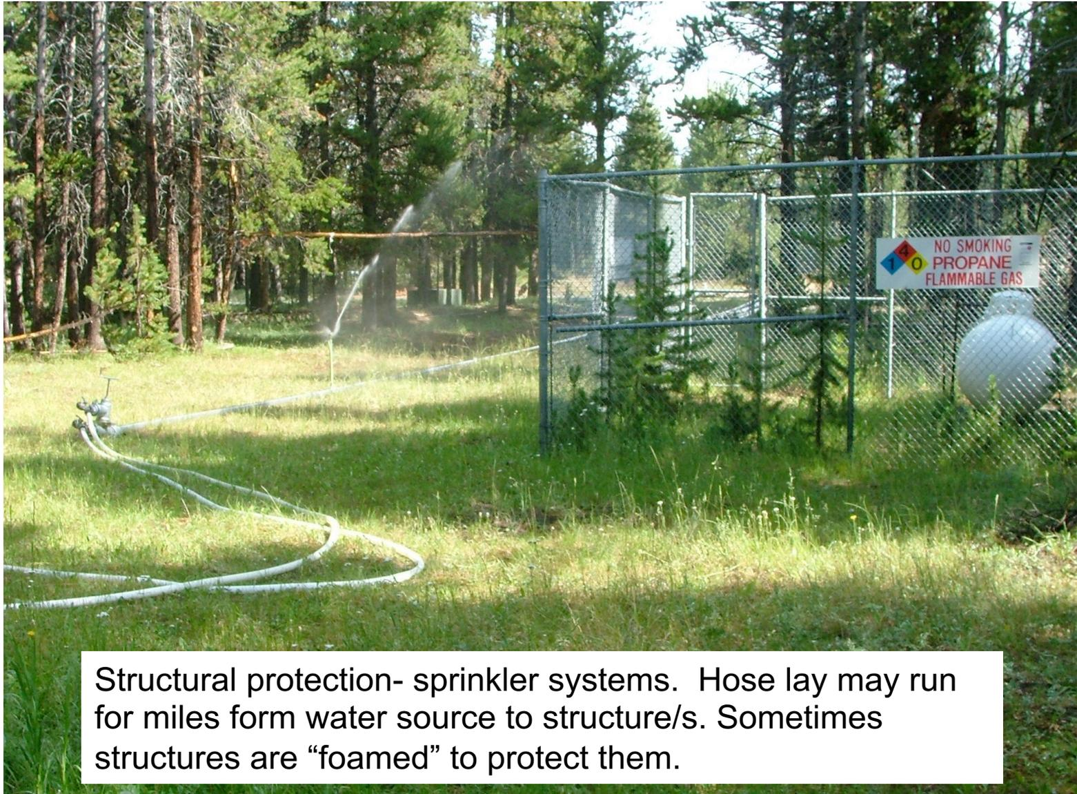
Structural protection- sprinkler systems. Hose lay may run for miles form water source to structure/s. Sometimes structures are “foamed” to protect them.
